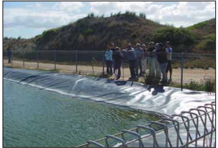
Recycled water storage
